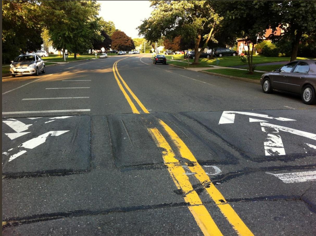
Humps like the one on Lake Drive at Valley Road do not accomplish the task because they were not built to standard dimensions.
